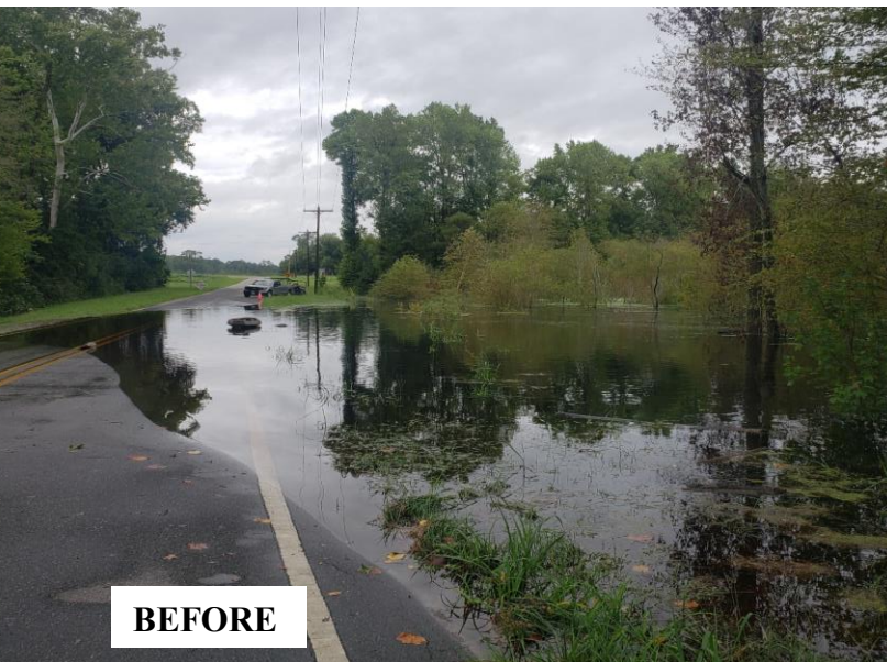
Austin Barnes, USDA Wildlife Services — Howell Swamp Church Road, Greene County, August 9, 2024. A beaver dam blocking the road culvert caused flooding on the road, threatening the driving public. BMAP professionals worked to remove the dam before Tropical Storm Debby arrived, preventing damage to the road infrastructure and benefitting adjacent landholders.
