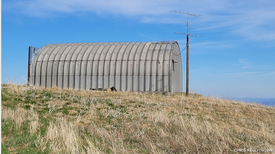
The Pond Mountain Motus Station in Ashe Co, NC. Antennas are mounted on a wood utility pole and the station's battery is charged by a solar panel. The receiver box and battery are housed inside this old airplane hangar.
