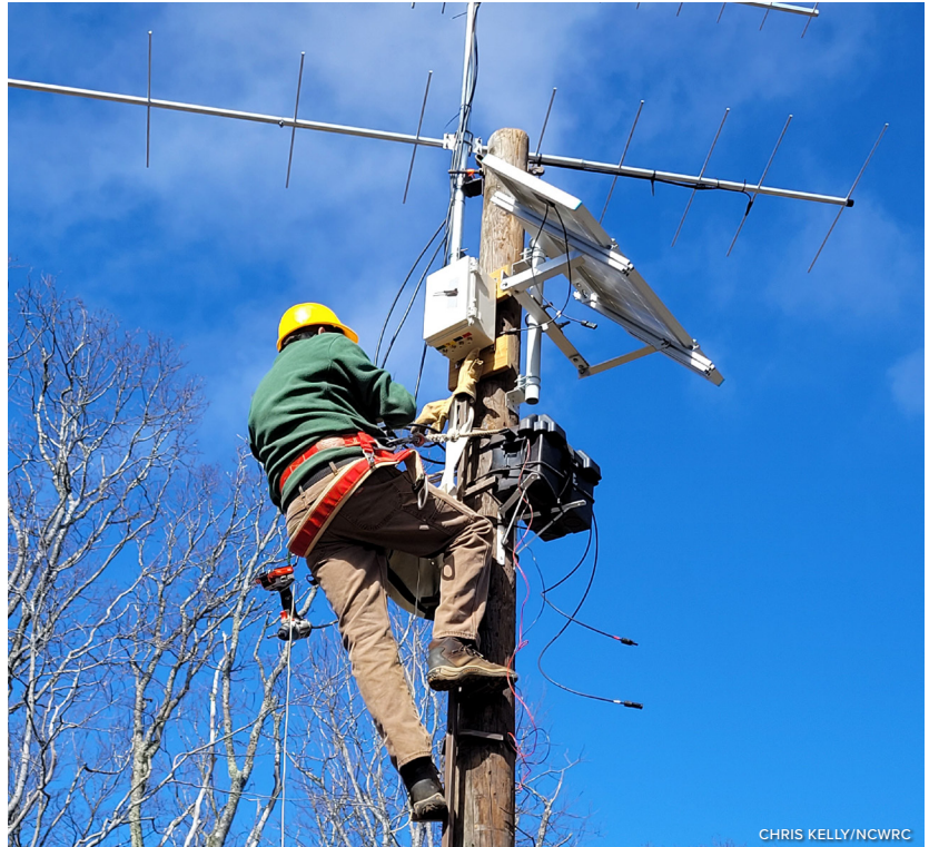
Kendrick Weeks connects the antennas to the receiver at WH Silver Game Land. The battery and charge controller are housed inside a battery box, mounted on a shelf bracket. The solar panel has its own mast.
